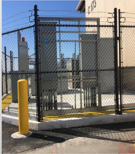
T-91 Substation Upgrades
